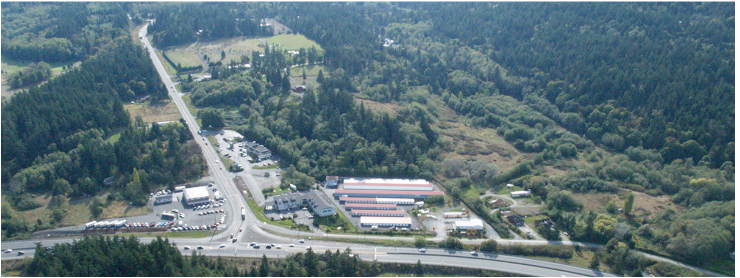
An aerial view of Sharpes Corner looking south toward Miller/Gibraltar roads.
